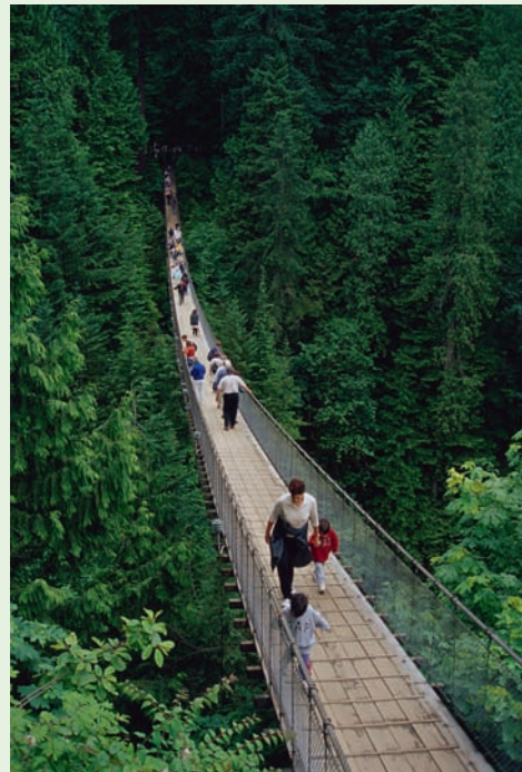
Figure 10.6 The Capilano River bridge
